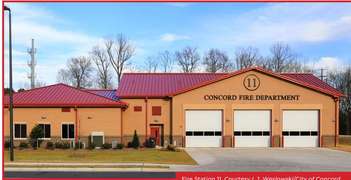
Fire Station 11. Courtesy L.J. Weslowski/City of Concord.
